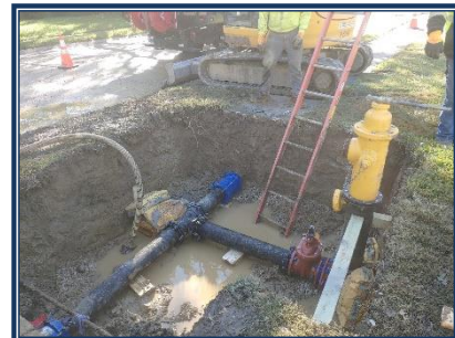
Hydrant Replacement on Woodgate
