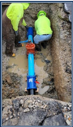
Valve Install on Lockett
