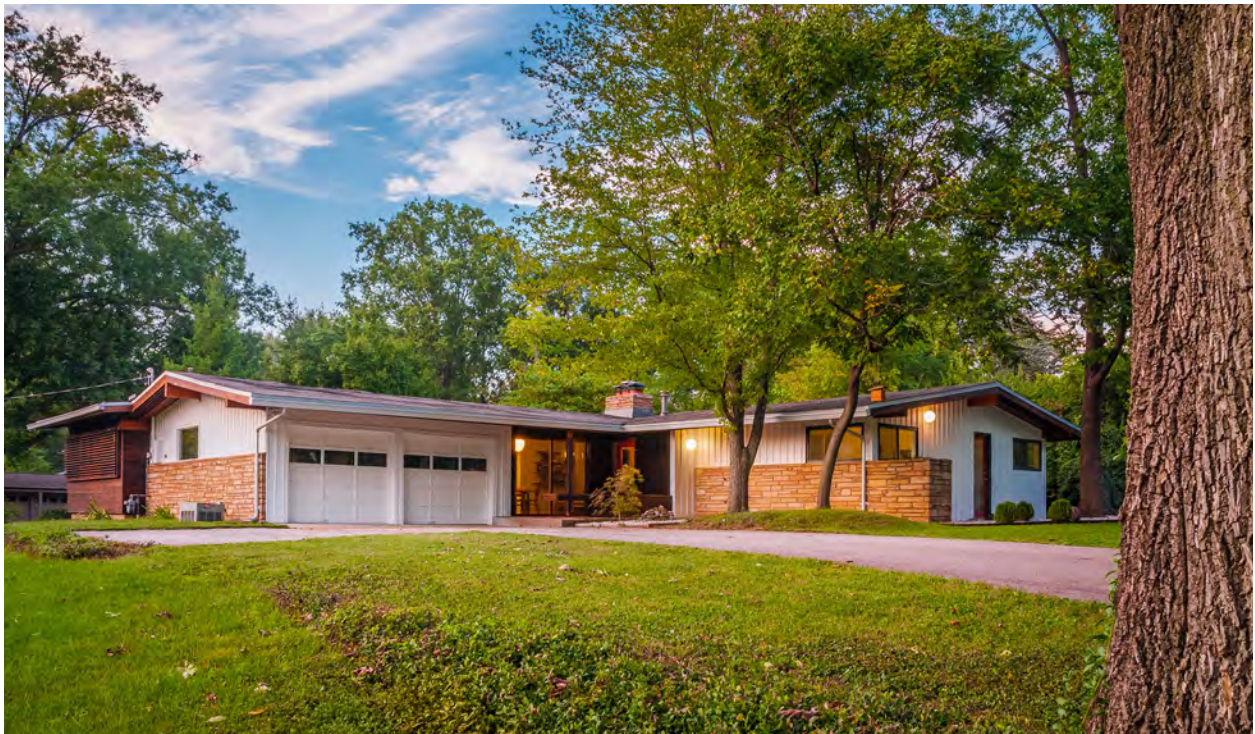
House at 1415 Lark Avenue photo credit Matt Marcinkowski
