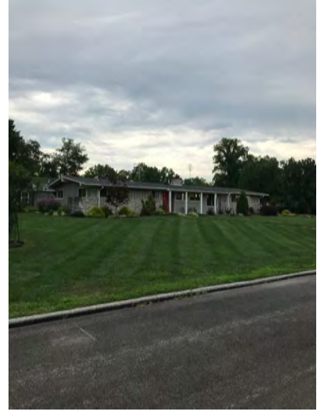
Examples of 'rectangular' floor plan houses at SCR. All plans feature low sloped roofs and extended overhangs, but have different garage configurations, different column treatment, and different masonry accents.
