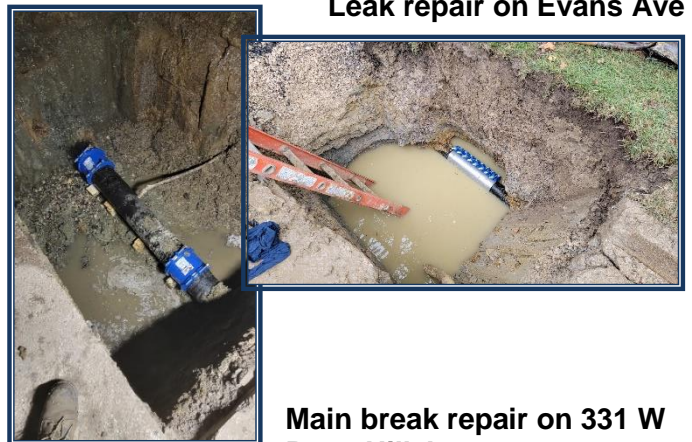
Leak repair on Evans Ave
