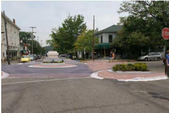
Miniature roundabout and curb bumpouts Photo by: Dan Burden, www.pedbikeimages.org
