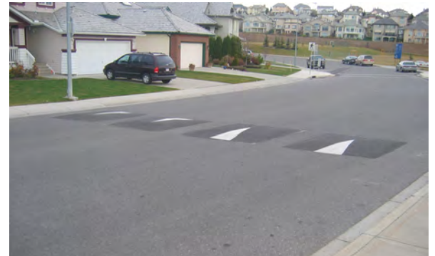
Speed cushions for designed for emergency vehicle access Photo by: Dan Burden, www.pedbikeimages.org
