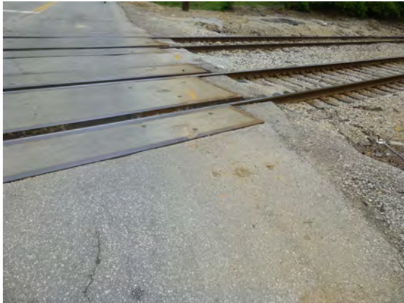
Gaps between the roadway and rail can pose a danger to people walking, biking, or using mobility devices.
