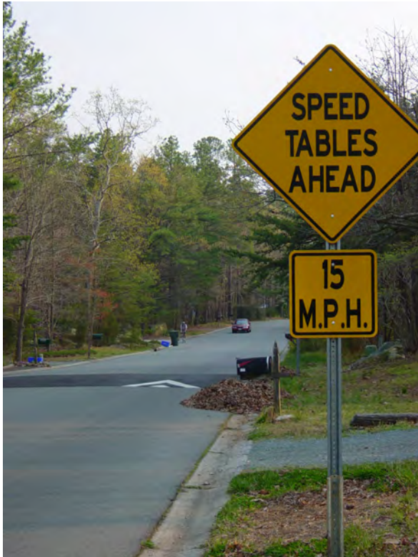
Speed tables are an effective and low cost traffic calming solution. Photo by: Austin Brown, www.pedbikeimages.org .
