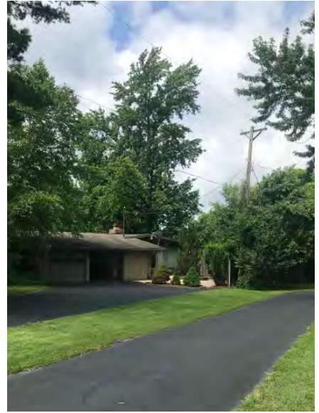
Public spaces in the houses have large expanses of glass that often follow the pitch of the low-sloped roofs. Also note the expressed beams on the exterior.
