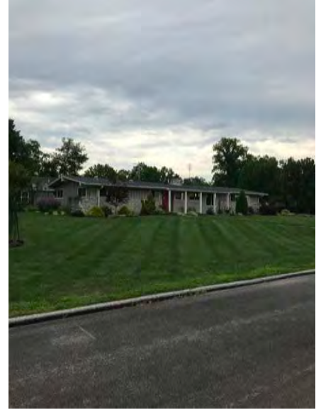
Examples of 'rectangular' floor plan houses at SCR. All plans feature low sloped roofs and extended overhangs, but have different garage configurations, different column treatment, and different masonry accents.
