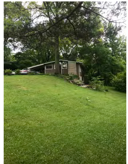
Example a walk-out floor plan house at SCR. These plans retain the single-story massing and appearance of the slab-on-grade ranch houses but use the sloped topography to incorporate walk-out basements.
