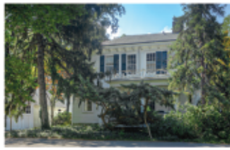
13. Murtfeldt-Douglass House 10 Douglass Lane
