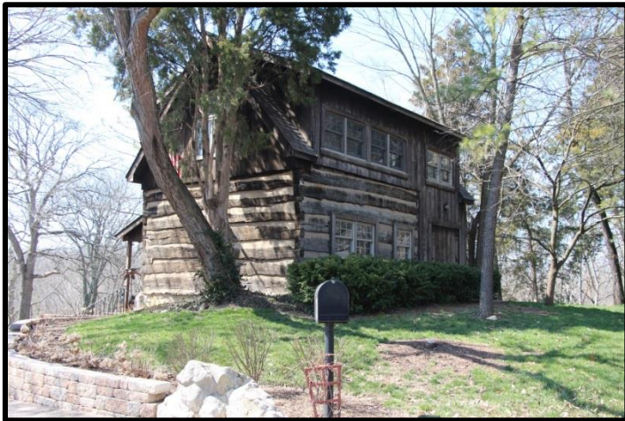
This is actually a log barn
