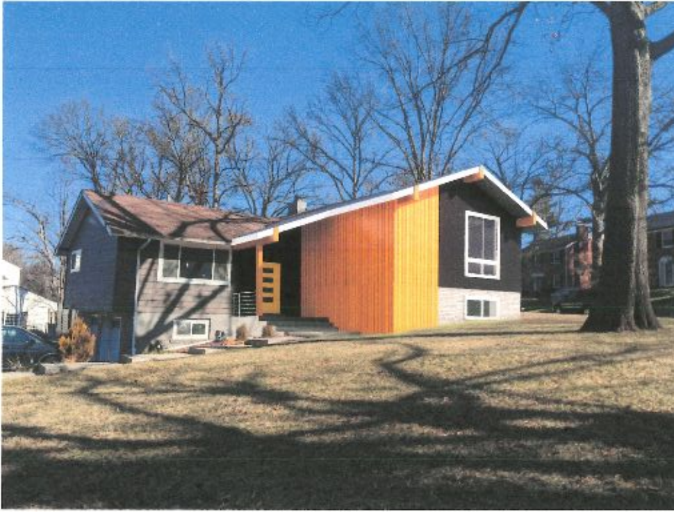
View from E. Glenwood Ln.
