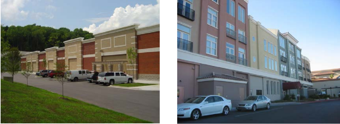
Figure 57-N: Illustrative example of two methods of using architectural features to create wall surface relief on wall elevations that are not the primary elevation.
