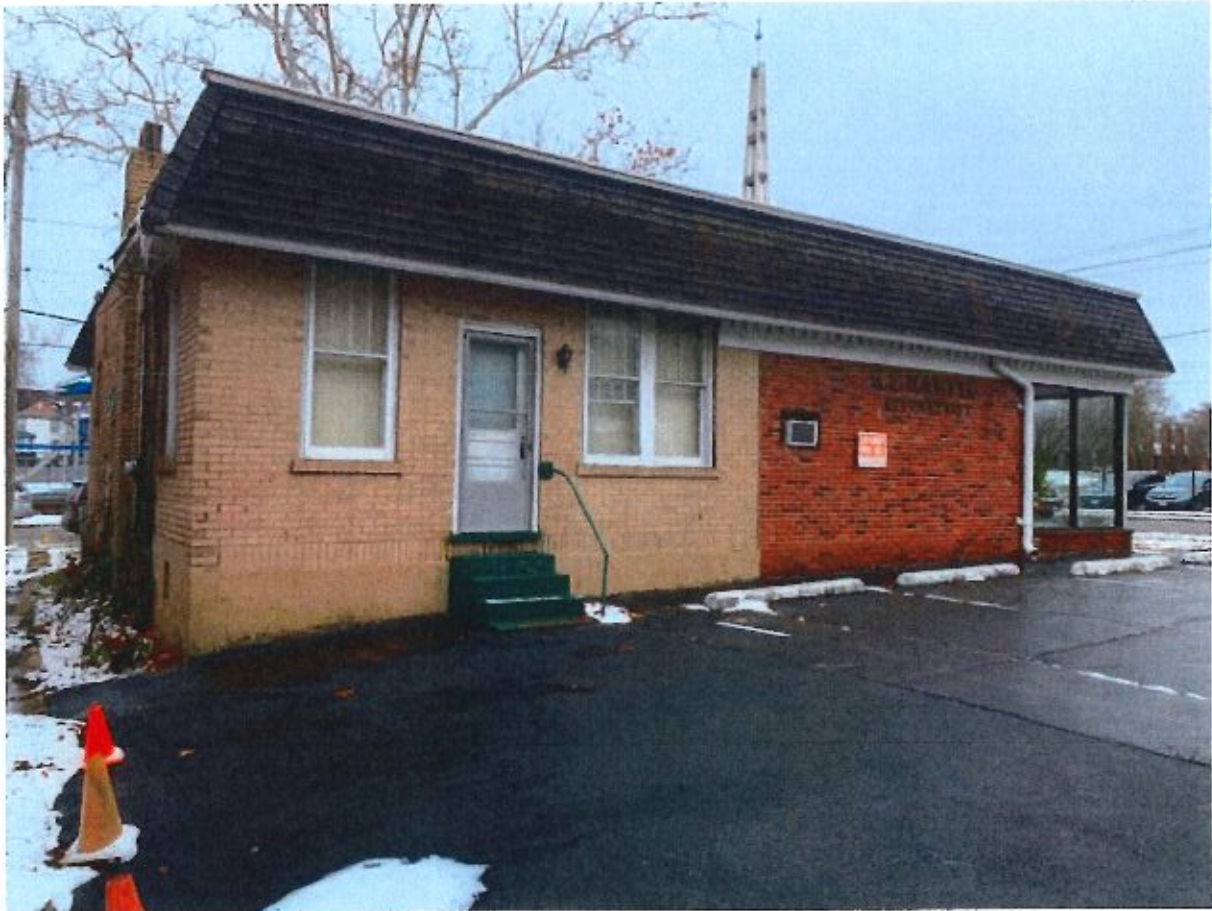
View of the east elevation of the existing building, taken from the existing parking lot, looking west
