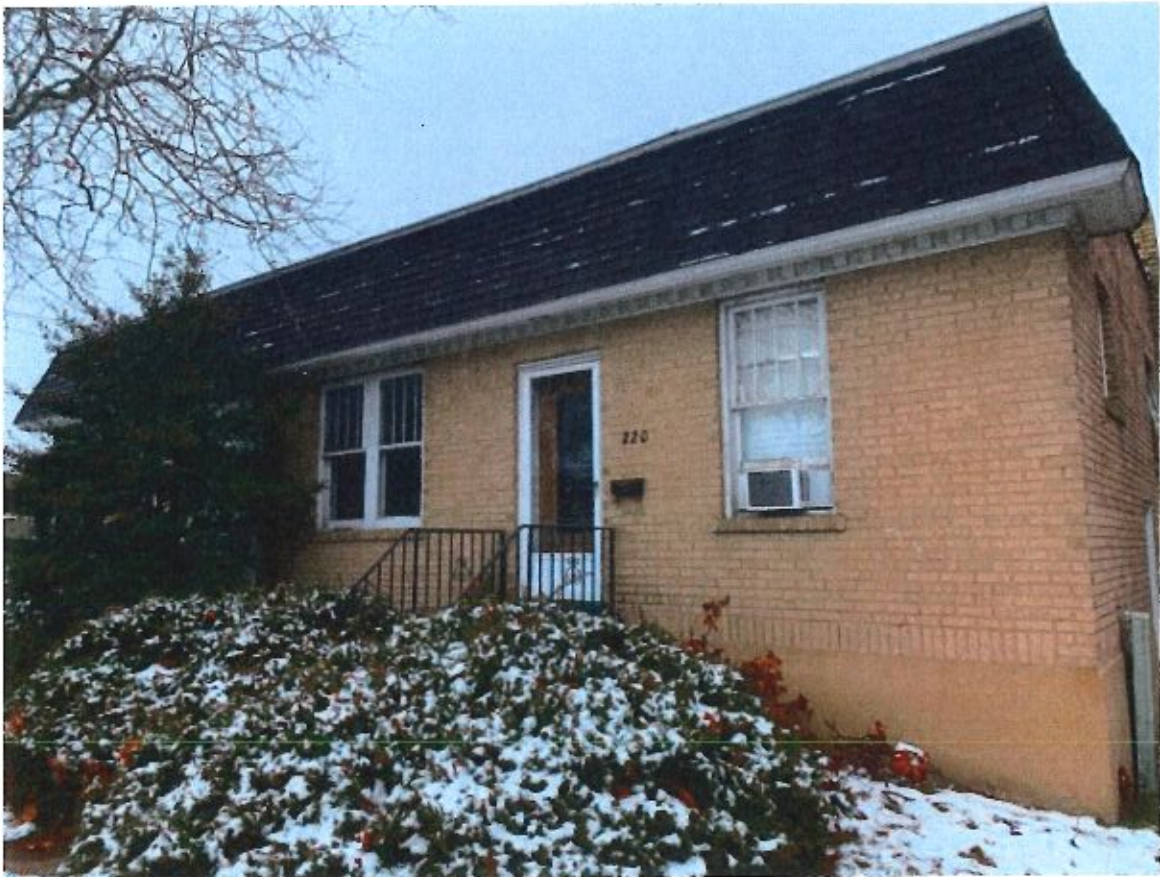
Close up of SWC of the existing building
