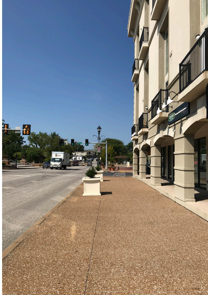
An opportunity for streetscape enhancement in order to create a more comfortable environment for pedestrians. Street trees or benches could create a buffer between pedestrians and vehicular traffic.
