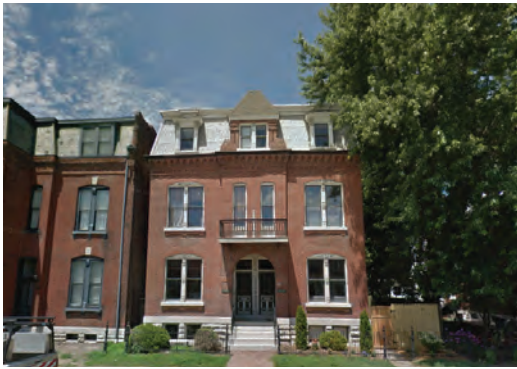
12th Street Mansion Apartments
