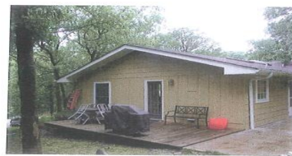
South Side & Rear Corner
