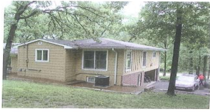
North Rear & Side Corner
