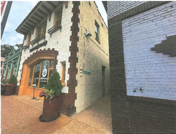
Adjacent Property to West
