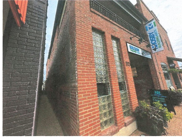
Adjacent Property to East
