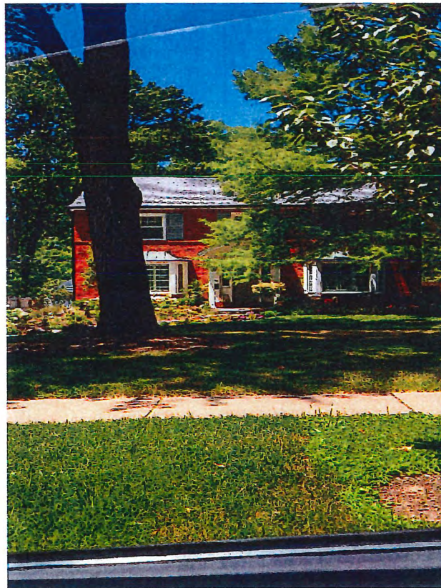
741 NORTH TAYLOR (ACROSS STREET)
